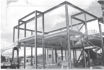
Typical steel framework.
